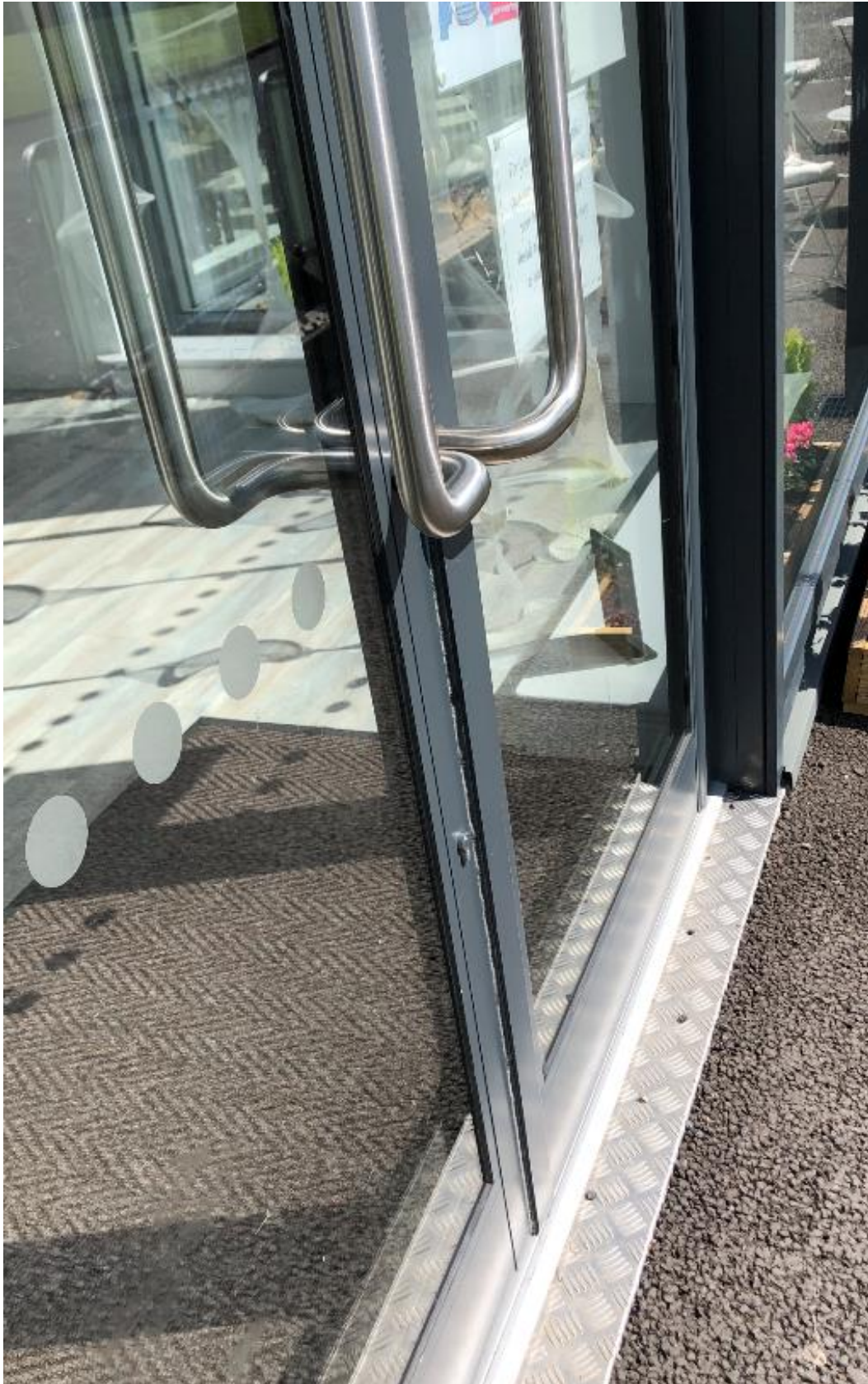
Photo 7 : Door, with brush seals showing
